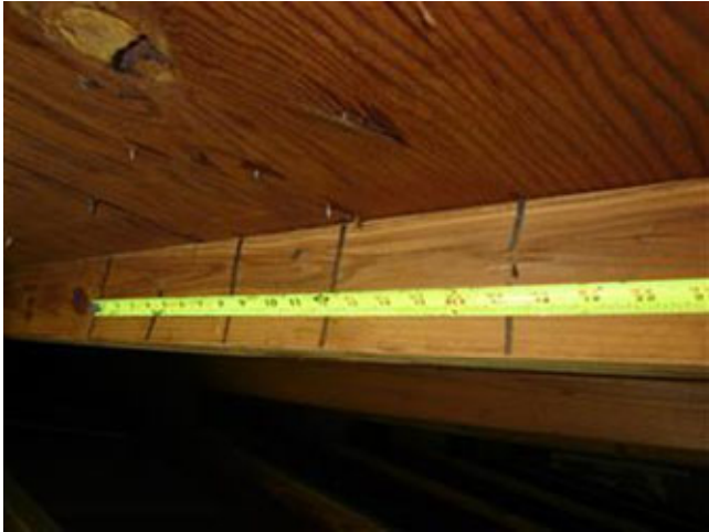
8d nails on 6" spacing
